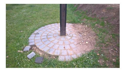
The dark patch is my footprint which covers a set of bricks which had broken loose. I commissioned Multibuild Construction, the builders who had constructed the plinth, to repair the damage and to add a retaining wall at the rear to restrict debris from the bund falling onto the plinth. This work was carried out in July/Aug and the plinth was fully restored.
