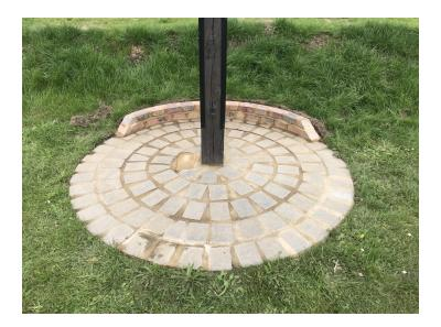
The bricks were attached using an industrial strength adhesive and pointed using the original cement mix.
